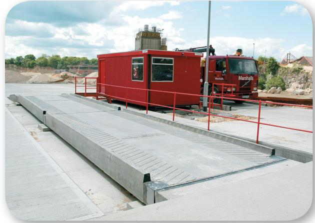
A weighbridge with steel fabricated structure is faster, easier and in most cases more cost effective to install. With a blast-cleaned surface and good quality painting, the steel structures can provide a hard wearing finish against corrosion and hence a longer life. These are also easier to relocate, if required.
